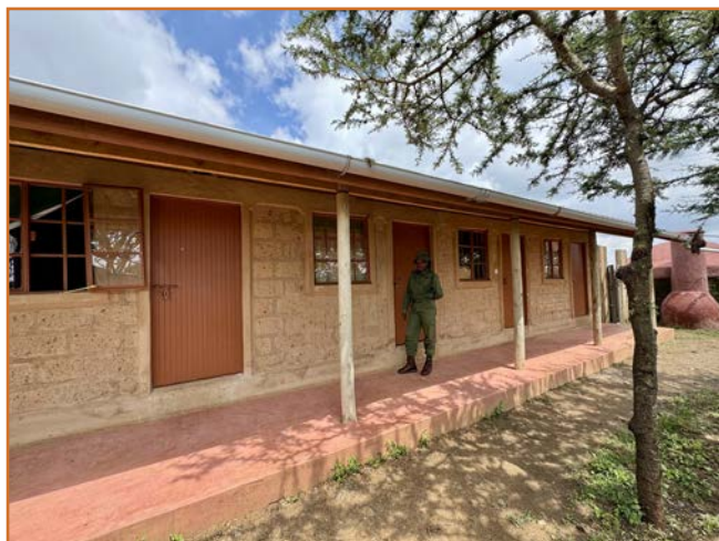
NEW RANGER ACCOMMODATION AT BRAVO GOLF
